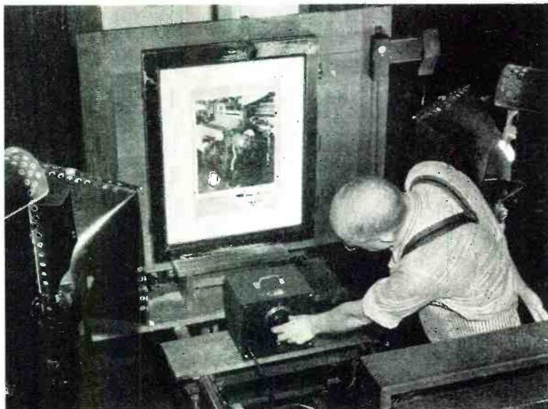
Photographic engineer using a Totalux to integrate light intensity with time, in reference to exposure in photography.
