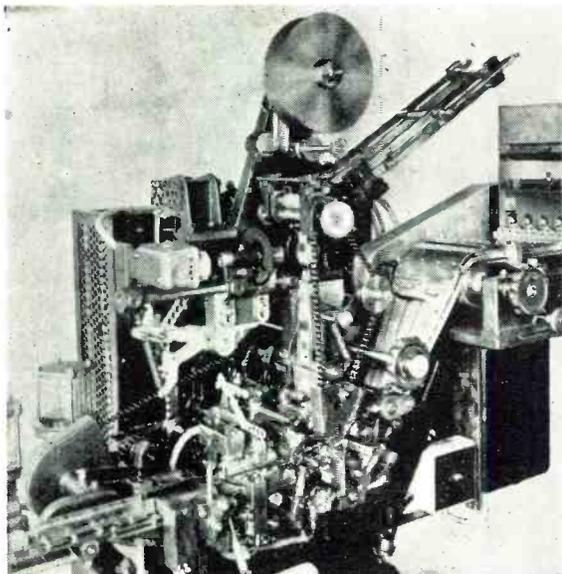
Cellophane wrapping machine using photoelectric relay to synchronize cutting and printing.
