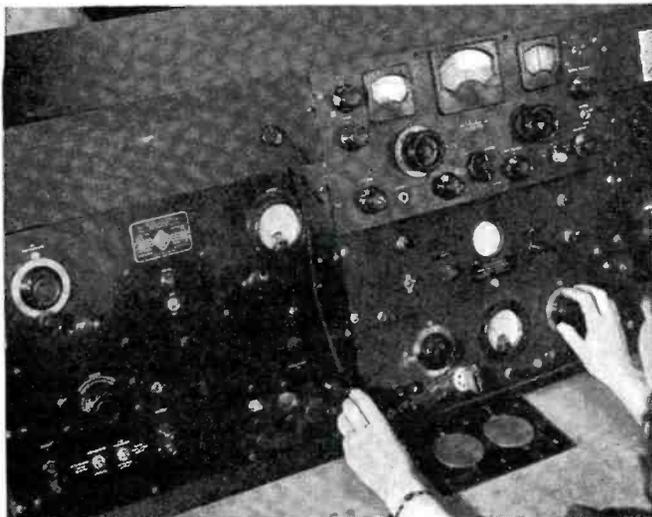
A channel sorter is used for rough frequency checks. The crystals are placed between the electrodes of the vise-like jig.
