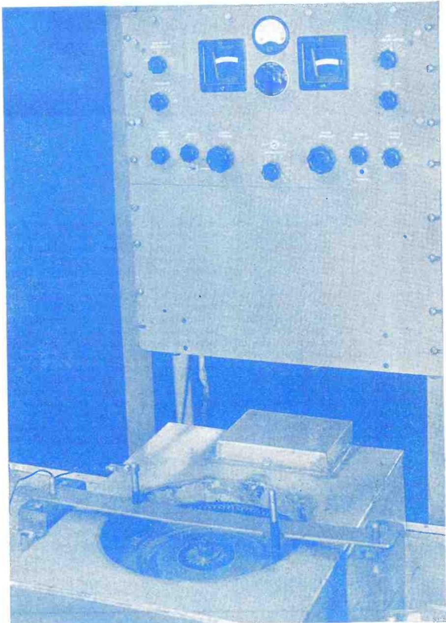
A quartz crystal lapping machine with a communications receiver for measuring the frequency of the signal produced by the crystals as they are lapped.
