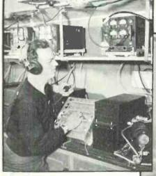
Picture shows technician checking electronic equipment for a F6F Hell-cat in the Communications Maintenance Laboratory aboard the Navy aircraft carrier, the "Shangri-La."
