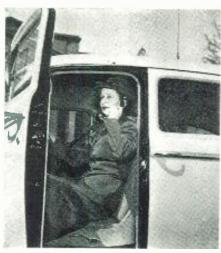
Woman taxi driver for the Yellow Cab Co. is shown using telephone handset in cab for test being conducted by the company in Philadelphia. Mobile two-way radio equipment installed in the test cab and a two-way "land station" on the roof of the 10-story Aldine Trust Building, permits conversations, reports, and instructions between the company's dispatchers and the test cab, whether parked or in operation. The antenna used for mobile operation is shown on roof.
