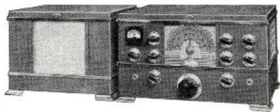
★ This is designed for the radio amateur and for general communications service in the 490 to 30,000 Kc. range.
