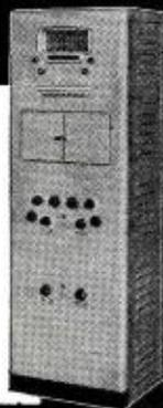
A completely pre-engineered system. Incorporates AM-FM radio tuner, record changer, controls, provision for wired music, and 90 watts of audio-power divided into four output circuits. Wired for optional remote control turret. Rugged all-metal cabinet with glacier-grey finish. Underwriters approved.
