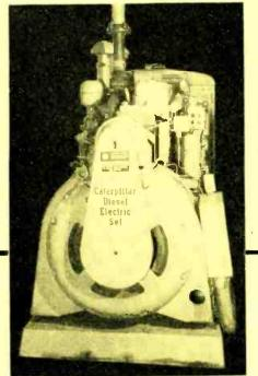
One of the Caterpillar diesel electric sets generating power for WOI-TV and FM transmitter at lowa State College.
