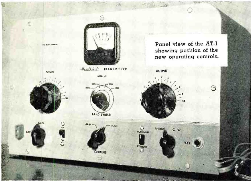
Panel view of the AT-1 showing position of the new operating controls.
