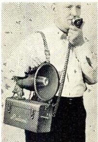
Microphone suspends from clasp. When not in use, is stored inside case.
