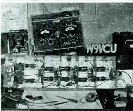
and two '58 tubes. The associated power supply to which it is connected by means of a cable and plug arrangement contains a power transformer a type 5Z3 choke and the condensers in filter arrangement. Two power supplies are mounted on this chassis, one for the sweep circuits and the other for the amplifier. The transformers are mounted along the rear side of the sweep circuit chassis and 2½ volt filament transformers are used to light all of the heaters in the transmitter.
