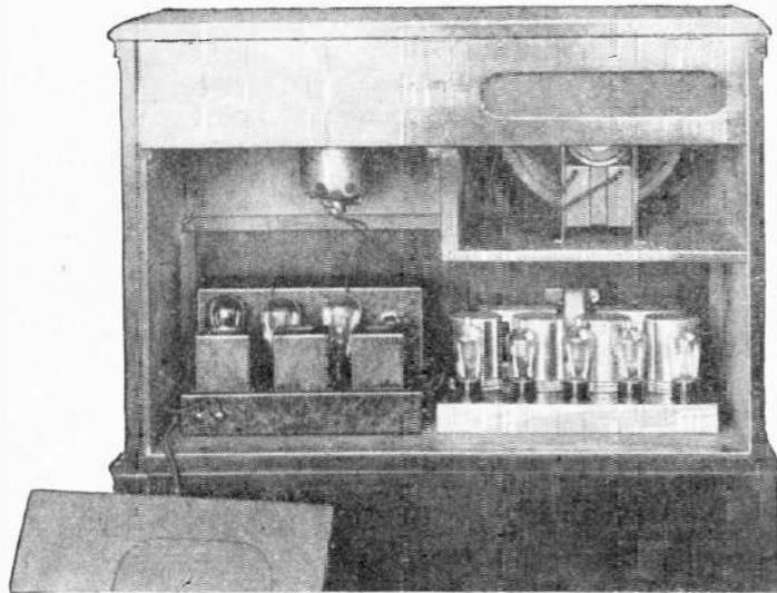
A rear view of the console cabinet housing the Velvetone tuner, "245" power amplifier, dynamic loud speaker and phonograph turntable
