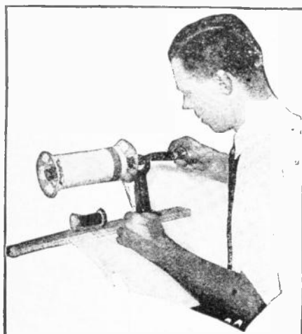
Better home-wound coils can be made when using some sort of winding jig, as shown. There is better chance of duplicating coils for matching purposes than if they were hand wound
