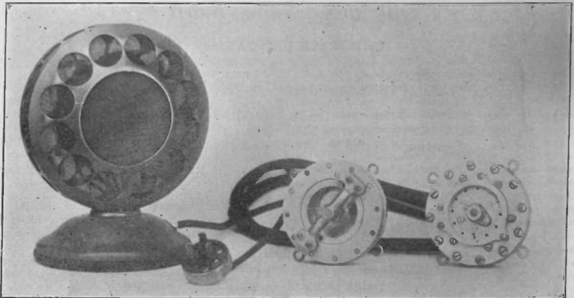
Fig. 2. How the Eaves-Dropper Looks When He Has Taken Off His Dress Suit. Front View in Middle, Rear View at Right
