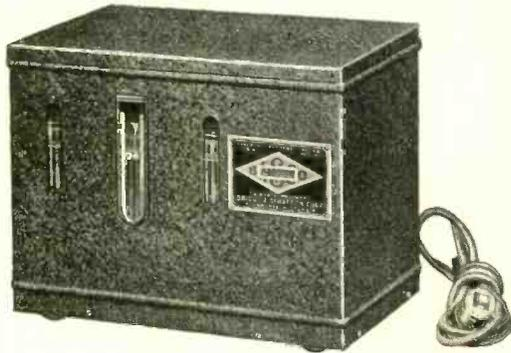
Basco "A & B" Unit. Entirely automatic in operation. Radio switch controls everything. Employs 45-ampere-hour Exide glass-cell battery, Raytheon rectifying elements, and Basco automatic charger. No line noises or distortion. Entire unit contained in compact, crystalline-lacquered steel case.
