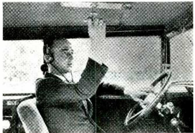
*A convenient arrangement which gives the operator control of the car, set and loop at the same time.*
