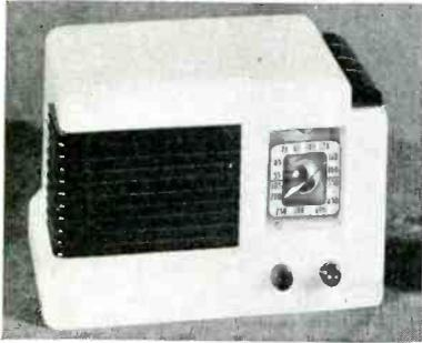
MODEL 551—Small table-type receiver with 5-tube superheterodyne; piano pushbutton tuning; with four color combinations of contrasting louvres and tuning keys; square shaped dial.
