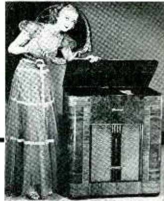
**PHONO-COMBINATION**—Model AK-59; 7 tube superhet with built-in antenna; 2 wave bands; push buttons for 5 stations; 12 inch electrodynamic speaker; tone control; Caphart record changer; provision for television; height 34¾; width 32¼, depth 16¼ inches.
