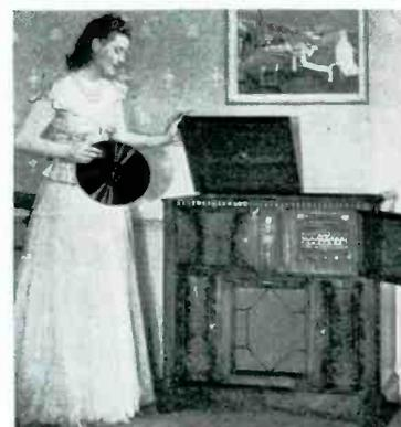
**RCA VHR-307** CONSOLE COMBINATION, a deluxe instrument, is available either in walnut or mahogany, incorporating radio, automatic phonograph, and home recording features. This 12-tube radio tunes 4 bands, including a special 31-meter spread band for ease of foreign tuning. Has a 15-inch speaker. RCA Mfg. Co., Camden, N. J.
