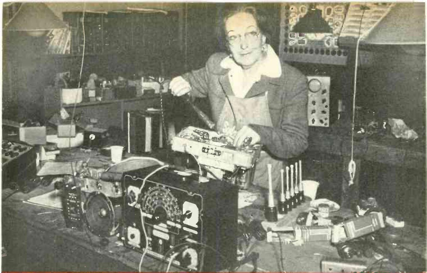
"Careful replacement technique involves good mechanical mounting of the parts and good soldering of joints to keep call-backs at a minimum," says Mary Wales. (Note ERT's Oscillograph Chart in background, Ed.)
