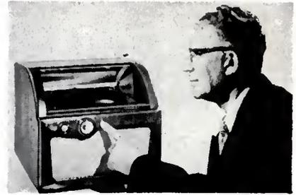
Edward Gray is shown starting his newly-developed Phono-Gard record player, which plays all 3 sizes of records without needle scratch. A transparent canopy isolates turntable and record, and the tone-arm moves from a locked and inaccessible position onto the record. No manual adjustment is necessary for record size. Player is excellent for demonstration playing and industrial programming.
