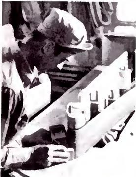
**EACH PIECE OF A CROSLLEY CABINET** is sanded at least five times—first by machine, and finally by hand with a paper so smooth you can't even feel its tiny grains!
