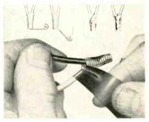
is snapped off. The electrical tape is started on the connector and brought forward to seal its bell end. Then, wrapped around the connector until it extends ½-in. beyond the small end of the connector, the tape is folded back and further wound toward the bell end to complete the splice. Minnesota Mining & Mfg. Co., St. Paul 6, Minn.—TECHNICIAN.
