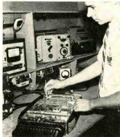
Technician nets receiver on frequency in the field maintenance shop.
