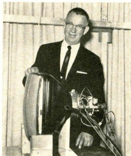
Elmer H. Wavering, president of Motorola, Inc., is shown with a 21 in. rectangular color CRT. The new addition to Motorola's color CRT line is being tested in a Helmholtz Chamber where the effects of magnetic fields in various parts of the earth can be simulated.
