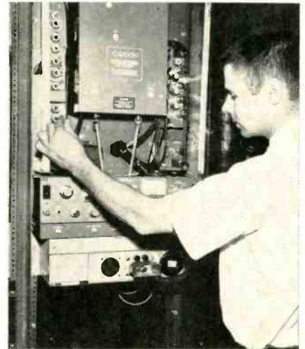
Adjustments being made on microwave station. This 8-channel system ties in remote base station sites in the upper parts of the county.
