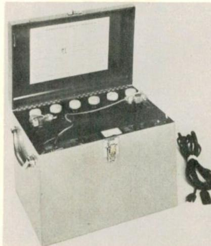
battery over the charging circuit. The recommended battery has a 55 amp-hour rating and is capable of storing approximately 660 watt-hours of energy. Of this, about 560 watt-hours are available at usable terminal voltage. Specifications include: output power, 140 watts max. continuous at 70-100% power factor, and 175 watts intermittent at 80-100% power factor for not over 15 minutes at 25% duty cycle. Cornell-Dubilier Electronics Div., Federal Pacific Electric Co., Fuquay Springs, N. Car.
