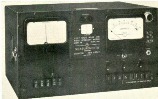
Measurements Corporation's Model 58-AS noise and field strength meter operates on 117 vac, 6, 12 or 28 v batteries.
