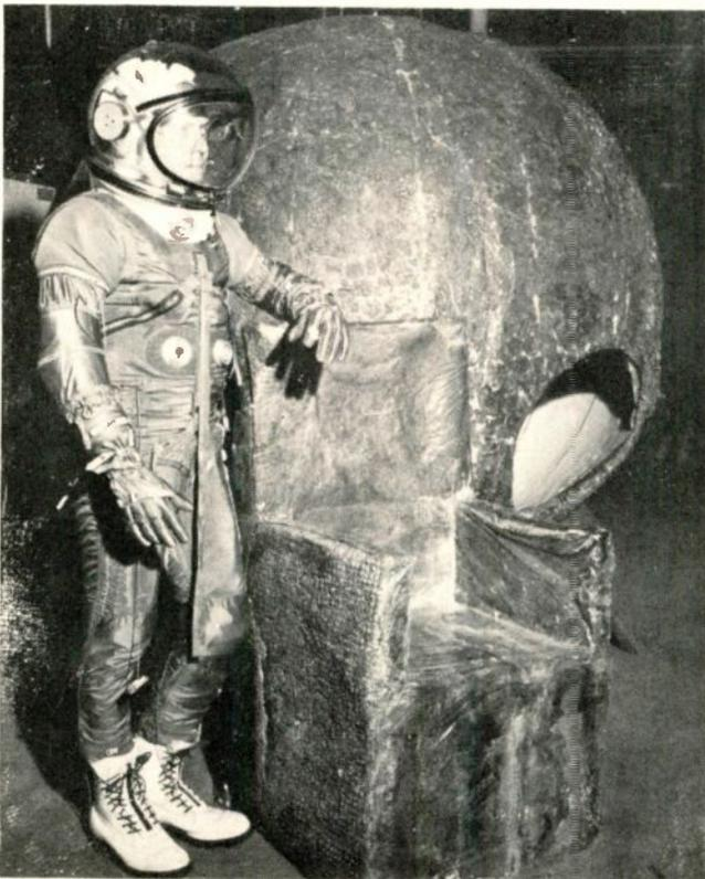
Space travelers of the future may have an easy chair and "igloo" similar to these which were formed from a new plastic foam material developed by Hughes Aircraft Co. for building light weight structures in space. Forms for the two structures were covered with thin discs that "sudsed" into a hardened mass after exposure to solar rays in a space chamber.
