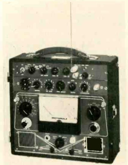
Motorola's two-way mobile test set, S-1059A, has built-in transistorized deviation meter.
