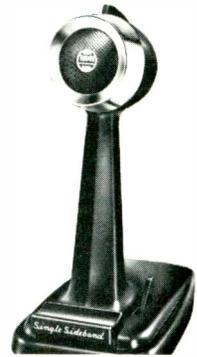
amateur use, is announced. A choice of PTT or VOX, 300 to 3000 cps, -48 db on the 454X crystal and -52 db on the 454C ceramic model, is available. Both microphones have a coiled cord as standard equipment. When wired for PTT, the 454 features two switching arrangements — push-to-talk, and a Lever-Lock switch to hold the microphone live. \$26.50 list, \$15.90 amateur net. Turner.
