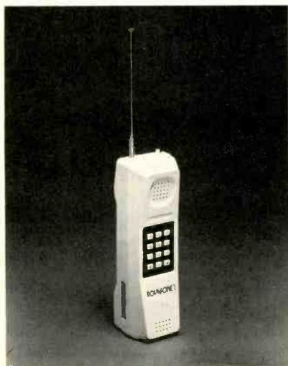
weighs 28 ounces and features touch pad pulse dialer, 16 digit memory of last number dialed, automatic redialing, and up to 40 hours of stand by time between battery charges. The system includes the base, remote, carrying case, 2 antennas, Ni-Cad batteries, remote charger, base power module and a modular line cord, and is approved for direct connection to a single phone line. The suggested price is \$649.95.
