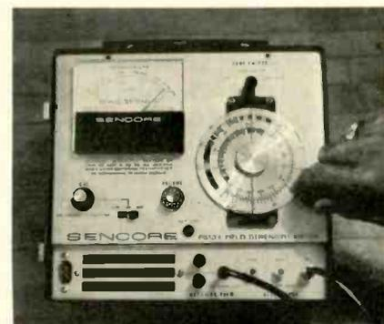
Sencore's Model PS134 Field Strength Meter was used to measure the antenna gain while adjusting the amplifier ZOOM control.
