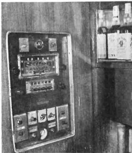
**Typical bar installation. Top panel has two speaker controls also magic eye, audio output-level indicator. A fine radio tuner with shortwave can be seen under controls. At the bottom are power switches, master amplifiers gain control, and the unusual, special remote reject and selector push-buttons for the record changer**
