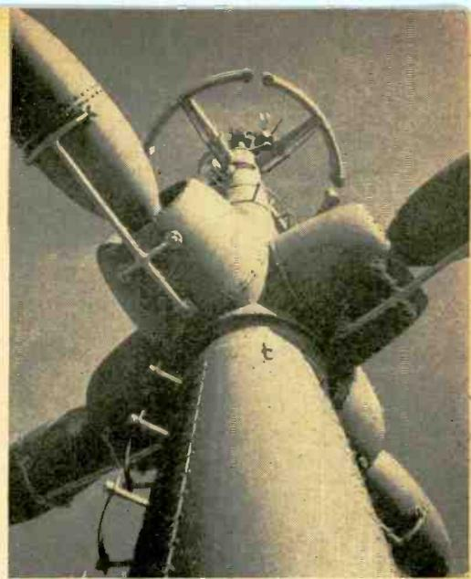
"Reaching" the market: Antenna of WNBT atop the 1280-foot Empire State building tower. Quadrants relay the audio portion of programs. Image signals go out from radial curved elements below.
