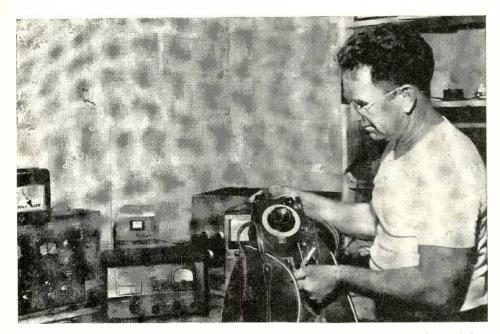
An accurate frequency meter is an essential piece of equipment for the mobile technician. One is shown here being packed in preparation for a service call.
