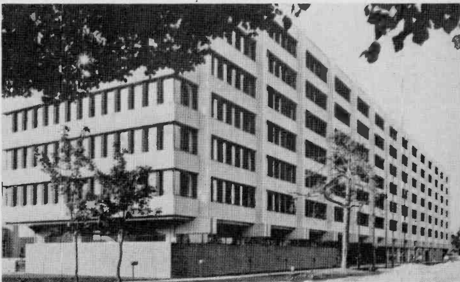
Since 1968 the programs of the Finnish Broadcasting Co. have originated from this modern building in Helsinki.
