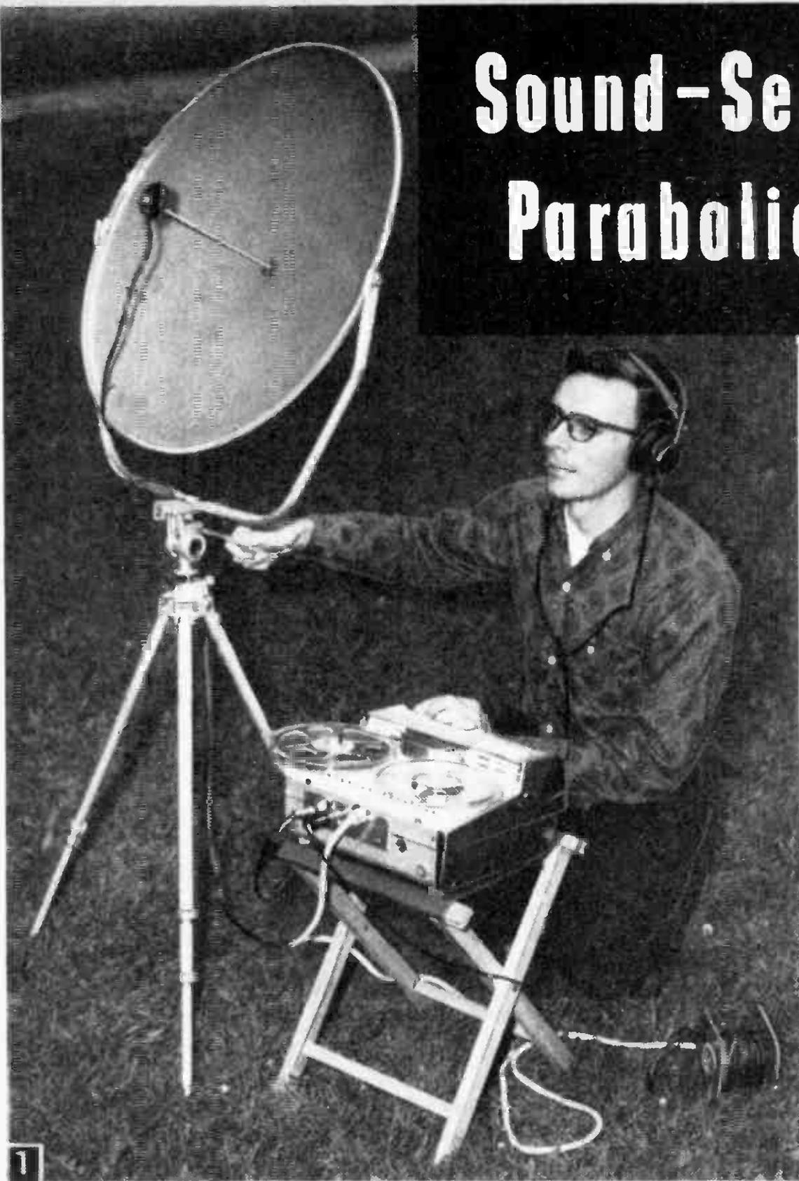
With earphones plugged into the output jack of a recorder, you can monitor the incoming sound. A disc (not shown) should be mounted in front of the mike to absorb unwanted sound.
