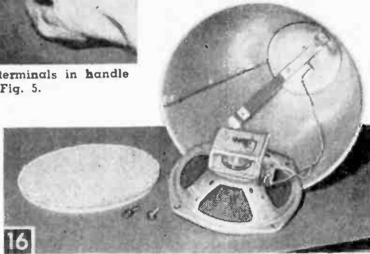
**16** Note speaker supporting U-bracket attached to wood disc at far end of horn. Speaker will mount against this bracket and grille cloth-covered wood ring at left will cover front of speaker. Note connected speaker leads going back through wood disc to amplifier.
