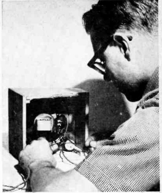
**NO BACK PANEL NEEDED!** Wire the L-Pad in place and just hang up. Wall behind baffle serves as back panel.
