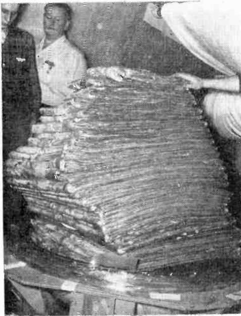
Echo II, comprised of some 54,000 square feet of specially laminated material, was folded and stacked, prior to being inserted by engineers into an 11-cubic-foot canister.
