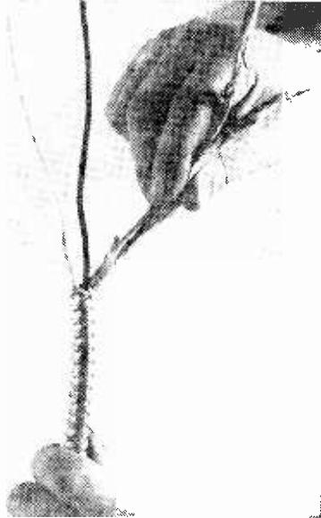
Remove kraft-paper wrap but not ground lead—bend back; wrap around cable; secure in clamp.
