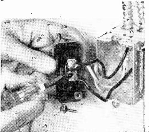
Soldered splices aren't used much any more. Circuit is completed by the connection between screw terminals.
