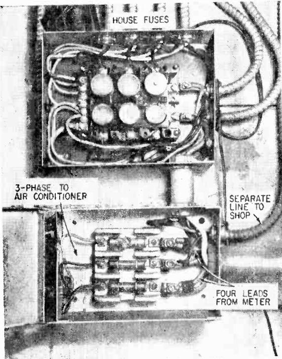
Removal of fuse-panel cover reveals details. Four wires from meter (lower right) indicate that service is full three-phase type. Big cartridge fuses in lower box are for air conditioner, top box is for regular circuits.
