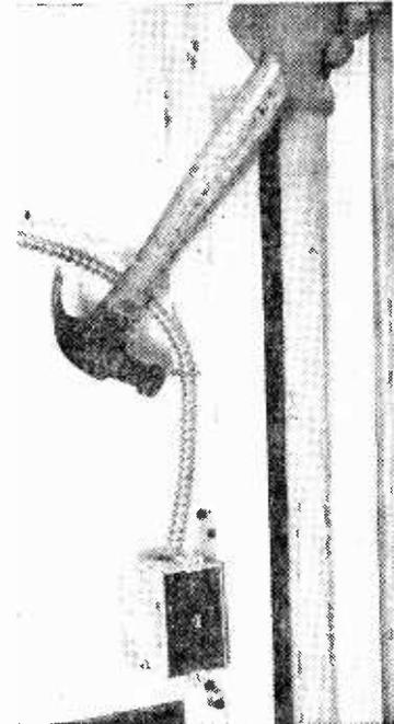
Last step is connection to circuit breaker. Wiring can't be live before; a safety step.
