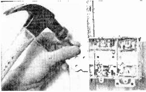
Special brackets make it a simple job to "hang" boxes for switches and receptacles. Hammer and nails are used by professionals for speedy installations while the homeowner will often use wood screws for less noise.
