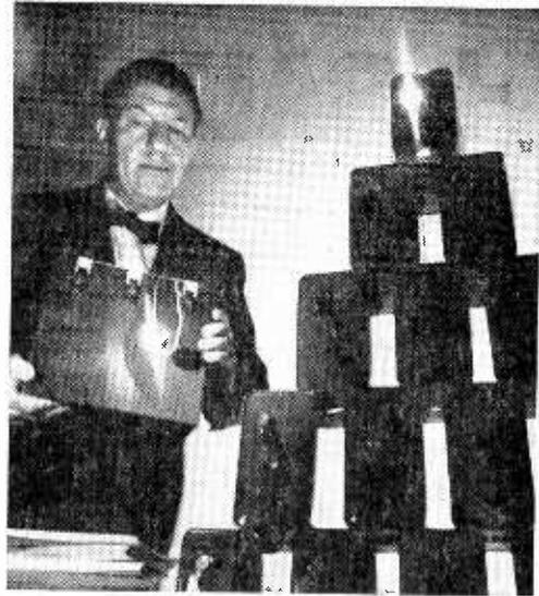
Single Magair battery packs as much power as stacked lantern batteries at right.
