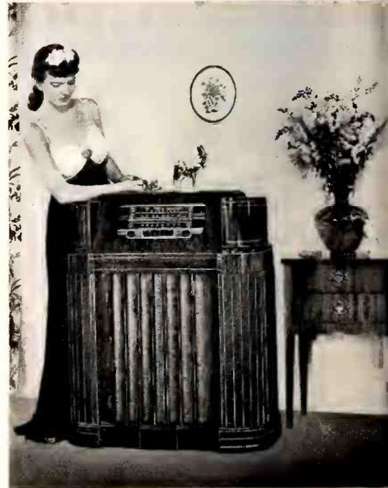
General Electric's console model LF-115, has 3 bands for FM, standard and short wave broadcasts. 11 tubes, 3 built-in beamscopes. FM Armstrong system.
