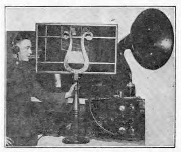
A loop antenna in the form of a lyre was displayed at the show by Corp.
