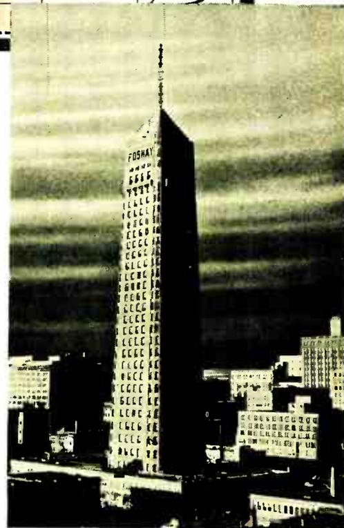
Federal's 8-Element Square-Loop Antenna dominates the ▲ Minneapolis skyline from the top of the Foshay Tower — highest building in the Northwest. Ruggedly constructed to withstand heavy winds and icing loads, this 80-foot antenna has already proved its dependability in temperatures down to 22 degrees below zero!
