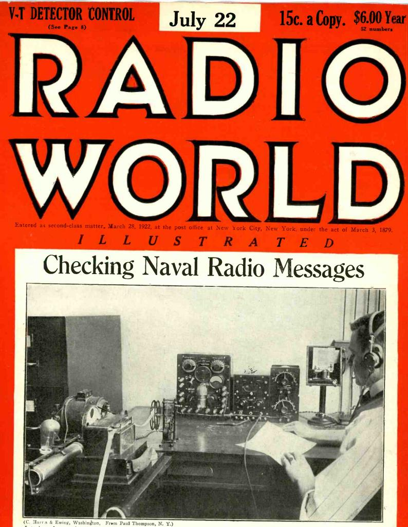
(C. Harrs & Ewing, Washington, From Paul Thompson, N. Y.) Interior of one of the remote-control stations of the United States Navy. This photograph shows no machinery for transmission—only the tape machine on the extreme left. Through local distance-wires dots and dashes are carried into the radio room of a distant transmitting-station. By means of necessary switches the operator can start the machine, which, in turn, broadcasts the messages. By this method all broadcast matter is checked up.
