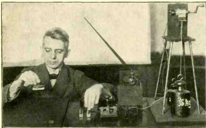
Fig. 1. Fundamental test of a new electrical phenomenon showing a metal plate clinging to a stone slab during the passage of a minute electric current.
