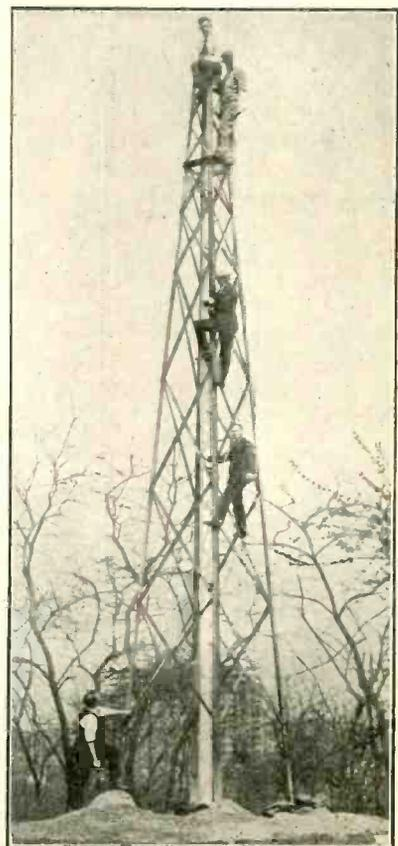
Located in a place which because of its surroundings did not permit the proper erection of an antenna, these members of the Radio Association of Greater New York built this 100-foot mast to get the best results out of their sets. The chief operator of the club, R. May, is seated atop the tower.
