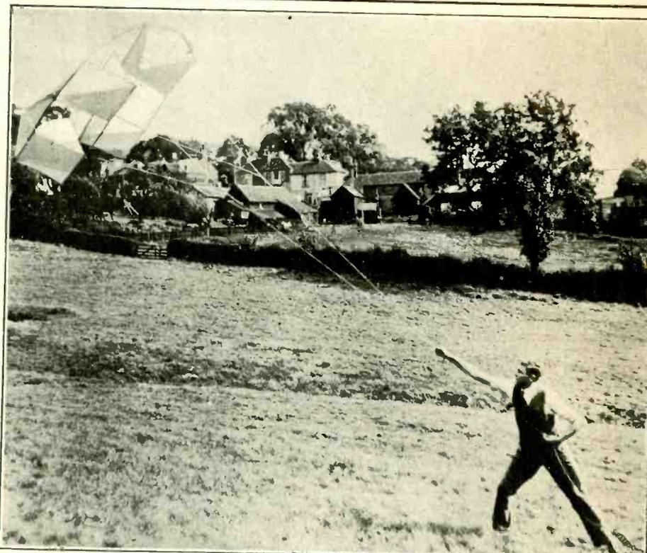
A HUGE KITE was used in recent tests at a radio field day in England for raising a long aerial to a position amid the clouds. A mobile station used the aerial for broadcasting. Note the insulator, at right, on the ground, showing where the aerial wire is joined as part of the kite string, and in this fashion raised. (International Newsreel)
