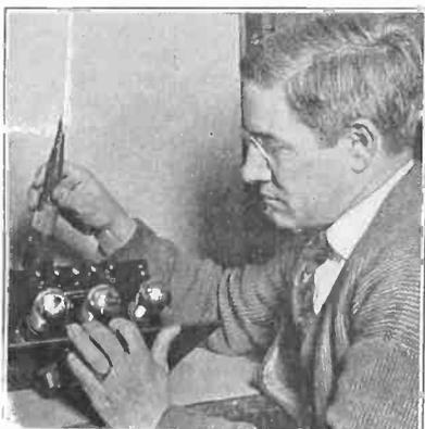
FIG. 1—Dust is injurious to any set, but especially in a Neutrodyne. The neutralization must be exact and is very critical. Dust increases the capacity of the transformer and is likely to throw the entire circuit out of neutralization. Neutrodynes when out of neutralization are uncontrollable in their oscillation. Keep the set in a tight cabinet, and dust thoroughly at least every six months.
