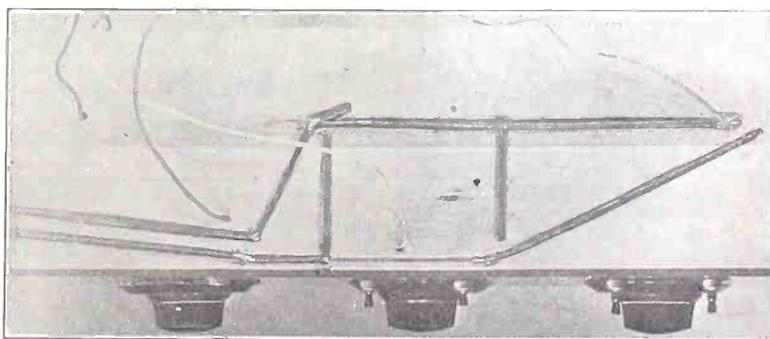
FIG. 5, an excellent view of the bottom of the set. Note the filament leads, identified by the heavy black leads. For the filament wiring use No. 14 insulated wire. Also note the leads coming through the holes in the baseboard, which are connected to the various batteries. **DO NOT FORGET TO PUT TAGS ON THE LEADS, so that you won't blow out your tubes.**
