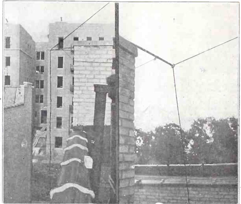
FIG. 3 (at left), showing how the lead-in should be placed. Note how far away from the building the wire is. Fig. 4 (at right), showing another view of the lead-in. Note the eyescrew at the end of the stick. Note how the antenna wire and
