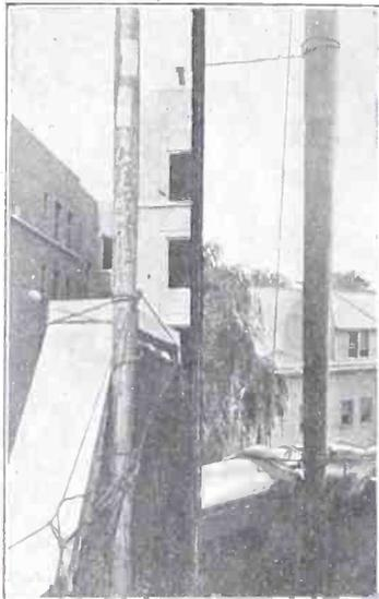
FIG. 1 (left hand photo), showing how one of the poles is held in place. This is at the slanting portion of the roof. Note the large amount of rope holding the pole. Fig. 2 (at right), showing how the poles which is at the cornice of the roof, looks. Note the guy wire coming down from the pole. The slot which is below the wire wrapped around the pole, was purposely left open so that you may observe what it looks like. Also note the peculiar middle section of the pole.
