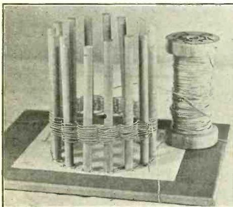
FIG. 8—The beginning of the winding process. No. 20 double cotton covered wire is used, being wound either in and out of every other turn, as shown, or in and out of every second turn. Both ways are equally good, the every-second-dowel shown, or in and out of every second turn.
