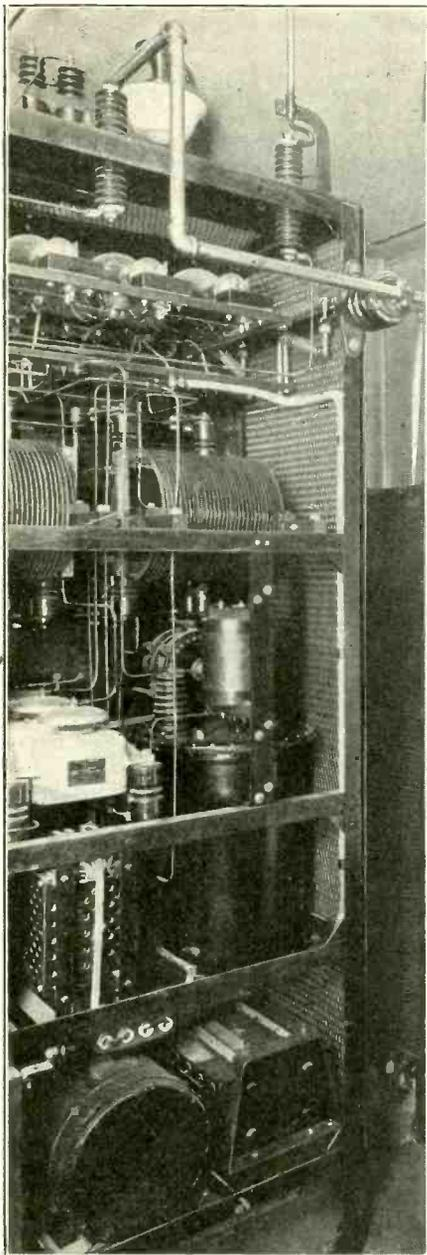
FIG. 4, the back of the 500-watt phone transmitter at WRC. Note the inductances in the fourth rack and heavy insulators on the top of the transmitter, also the large condensers in the third rack.
