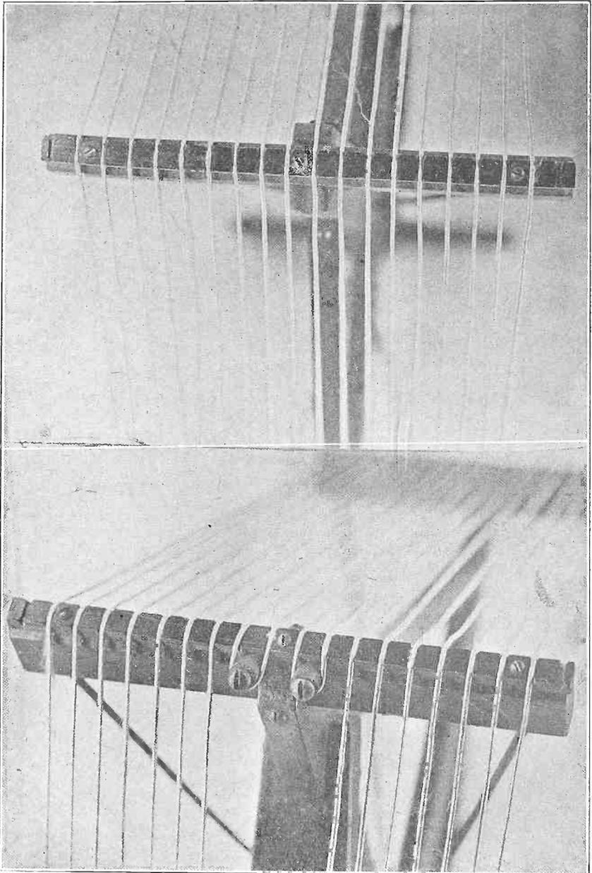
FIG. 8—After you have constructed the box frame of thin pieces of wood, cut four pieces of Bakelite 5" long by 3/4" square. Then file little notches 1/4" apart (20 in all) in these Bakelite strips, clearly shown almost full size. These are attached to the four corners of the box frame by
