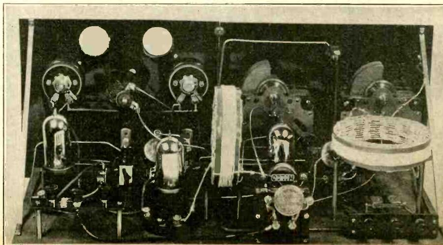
A 3-TUBE RECEIVER, employing a step of radio-frequency amplification, detector, and a step of audio-frequency amplification. The RF transformer and the detector coil are mounted to prevent stray coupling.
