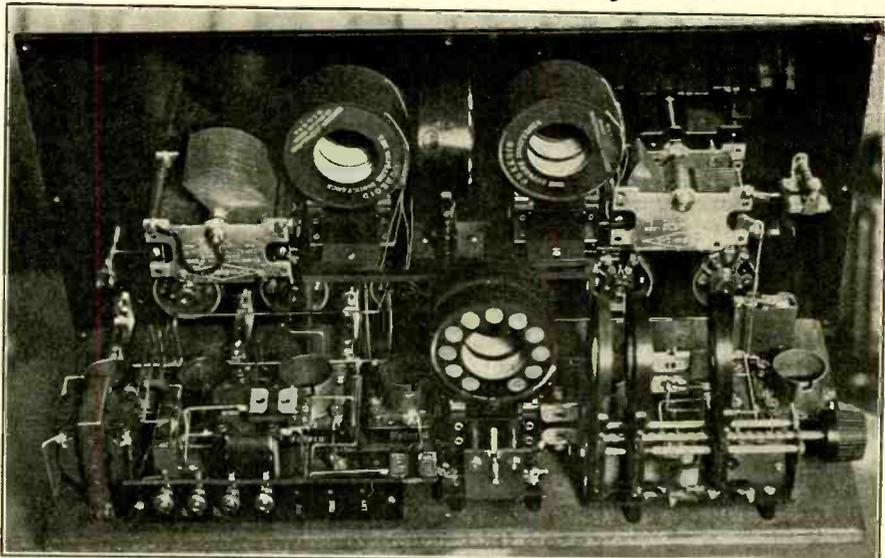
A 5-TUBE Super-Heterodyne, employing curkoid coils. The oscillator coils are at the right. The whole outfit is on a panel 16x3 1/2".
