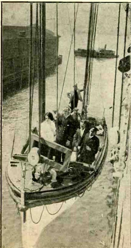
THE wireless-equipped lifeboat of the SS Orbita, the first of its kind being lowered over the side of the steamship. A directional loop is employed with this receiver to ascertain the direction from which rescue ship may be approaching. (International Newsreel).
