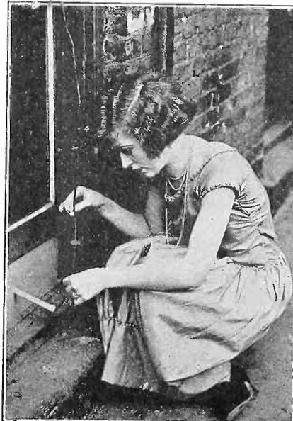
PUT a porcelain lead-in insulator at an angle pointing toward ground, so that water won't get inside your house or provide a leakage path for the radio waves. (Kadel & Herbert).
