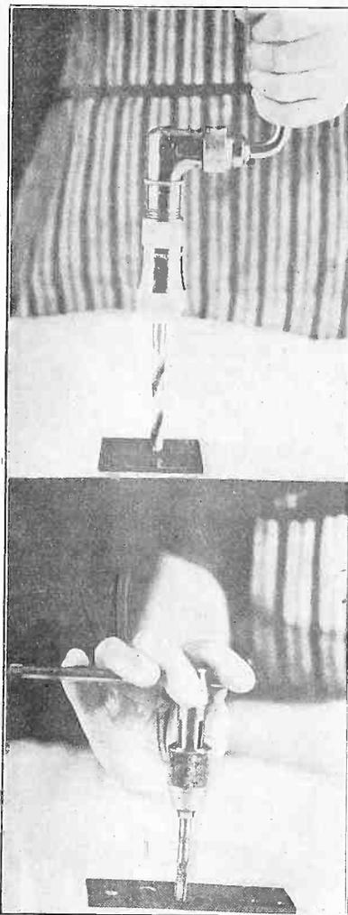
IN USING a twist drill, if the drill will not make a wide enough hole (top photo) then use a reamer, as shown in lower photo. (Hayden Studios).
