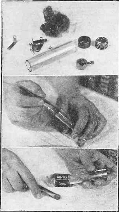
FIG. 1 (top). The parts required for making a fixed crystal detector are: One piece of steam gauge glass tubing; one crystal; small quantity of No. 00 steel wool; four clips for mounting; screws; two end caps taken from an old cartridge-type fuse. Fig. 2 (center). Fill one end of the tube with steel wool about half way. Fig. 3. Insert the crystal as shown.
