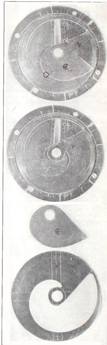
FIG. 8, the cams of an SLF dial. They are A and B. When B is superimposed on A an angle O is developed. In the slot (under shaft hole) a pinion moves up and down, depending on how you turn the dial knob attached to the pinion. The slot is toothed. If point O is brought down to the slot the pinion will move the circumference of A evenly, for dial readings, but, due to the shaped cam B, will introduce slow motion, or much slighter capacity change, on the lower waves.
