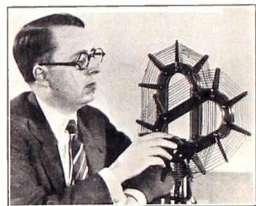
STEWART C. WHITMAN demonstrating his new tuning loop aerial. It is the first loop of its type that tunes the incoming signals to the peak of the wave desired. Tuning is simplified, in that all dial readings may be Calibrated. A great directional effect is obtainable with this loop. (Kadel & Herbert.)
